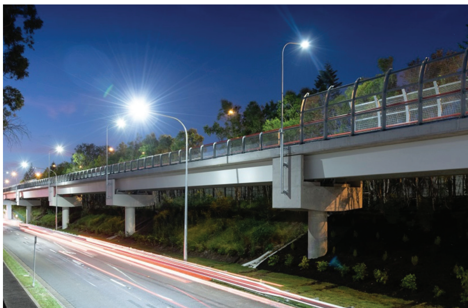
The NPA has asked the government to consider grade-separated, safe cycleways as part of the Warringah Freeway project to reduce traffic – similar to what Queensland is building (pictured). Image courtesy of Queensland Government, Department of Transport and Main Roads.
